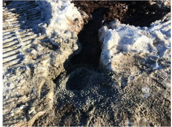
Photo #10 View at sealed borehole 1359-10 (1).
