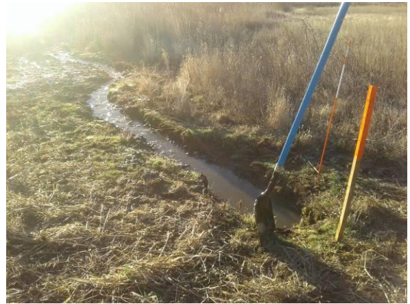
Photo #4 View of trenching at borehole 1359-10 (1).
